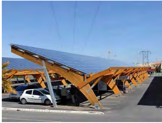
Figure 48 : Ombrière photovoltaïque
